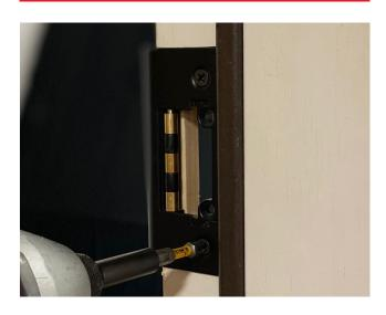
Retighten short screws to secure strike plate assembly at its adjusted position.
