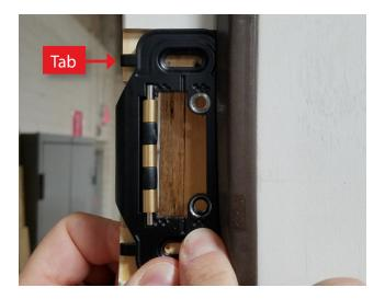
Place the reinforcing roller plate into the mortise and align the tabs shown with the edge of the frame. Use a rubber mallet to drive the cleats on the back of the plate into the frame.
