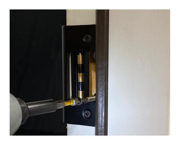
Place two of the longer 3" screws provided, through the two holes in the reinforcing roller plate.
