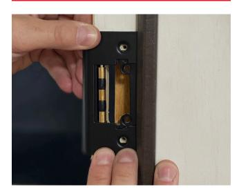
Place strike plate on top of reinforcing roller plate. Orient curved lip towards frame edge.
