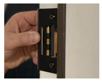
If adjustment of the strike is required to either loosen or tighten its fit with weatherstrip, first partially loosen short screws.
