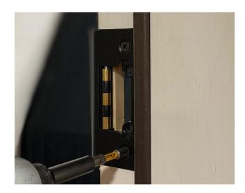
Secure the assembled strike plate with two of the provided 1/2" screws.
